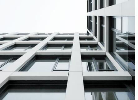
To secure non-visible fastening, an intelligent system with integrated fastening anchors was developed. Weather-proof pre-assembly in the factory guarantees a high standard of quality and rapid assembly on-site. The elements are simply hung into place and finely-adjusted into position.
