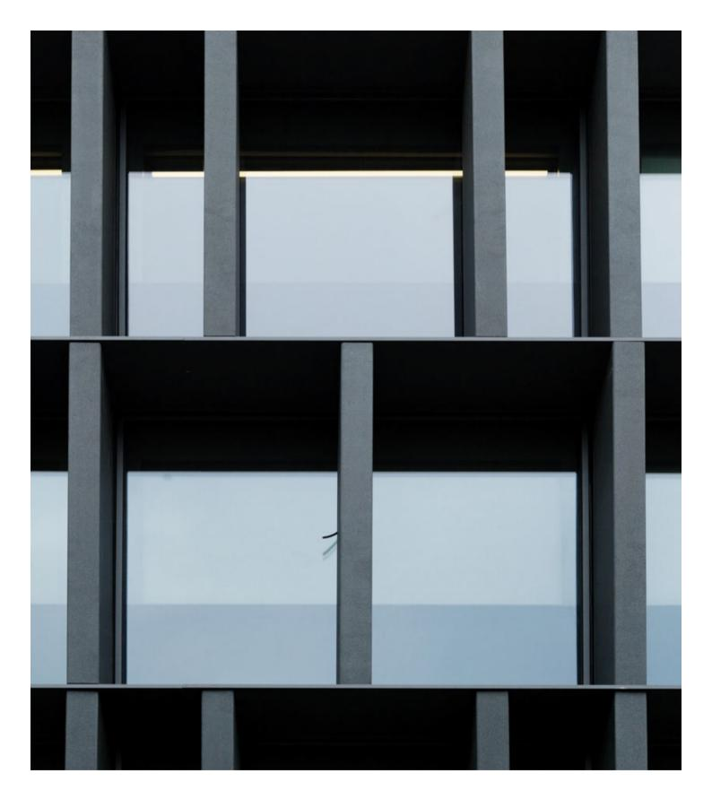
**formparts**folded glassfibre reinforced concrete panels for facades
