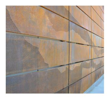
or-Ten steel is versatile and can be adapted to any building type and geometry. It can be utilised as an element in an exterior rain screen facade, within an interior panel system with a high performance clear top coat (or raw), as signage, or in artistic pieces.
